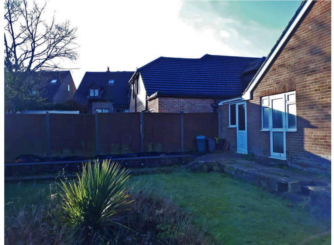
View to 80 Lower Buckland Rd
